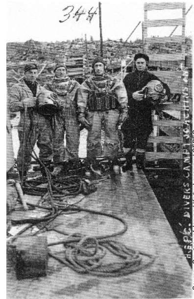
Figure 2.72 Divers Building the Dam at Rapides-des-Joachims
