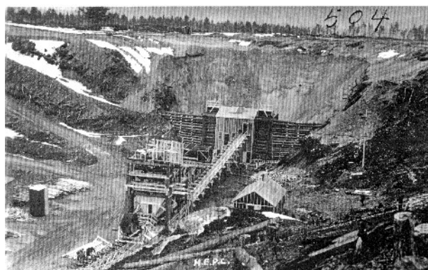
Figure 2.77 Building the Dam at Rapides-des-Joachims
